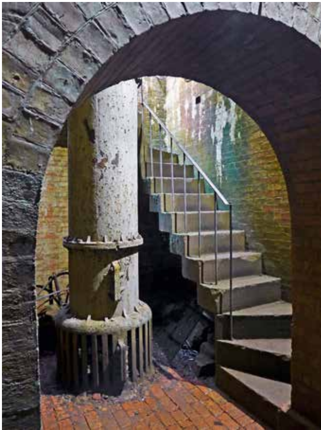
Papplewick Reservoir: Access Stairs. Photo Tim Wellburn
